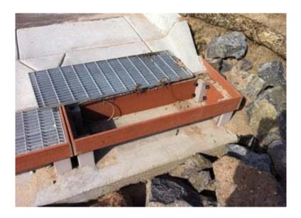
Rain Guardian placement and methods of routing water to the chamber are highly flexible and can therefore easily accommodate site-specific conditions (e.g. utilities and sidewalks).
