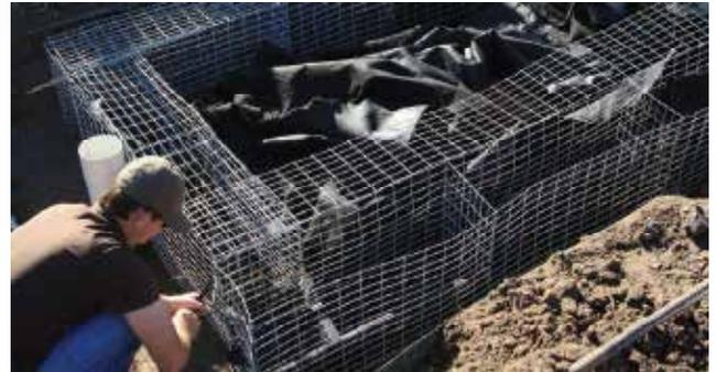
Figure 24: Place gabion wall so that it is square and level
