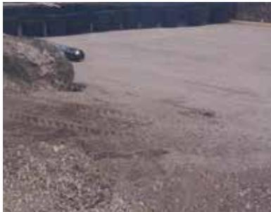
**TIP:** Creating a smooth, level platform will allow for faster installation of Modular Underdrain, as units will fit together evenly, eliminating detail work that can delay your progress (Figure 5)
