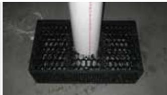
Figure 13: Place inspection port into underdrain module
