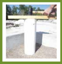
Figure 3: Hammering Pipe Into Media
