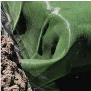
Fold Mesh for outside corners similar to sheets on a bed, and lay excess material flat against Modular Underdrain. Leave corners loose to avoid creating weak spots in the material. Temporarily secure excess fabric with duct tape (Fig. 17 left).
