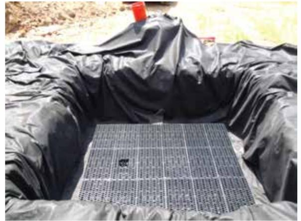
Figure 8: Place modular underdrain in specified configuration within geotextile envelope.
