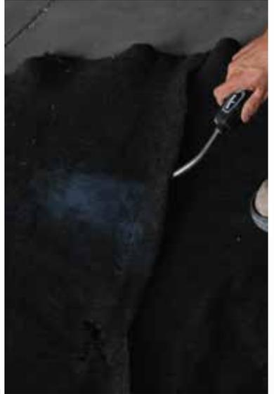
Figure 29: Geotextile being melted together with a torch.
