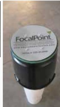
Figure 14: Cut inspection port to appropriate height stated on plans. Seal the opening on top of the pipe with the FocalPoint Inspection Port Cap or temporary lid
