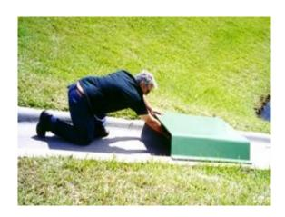
Step 1: Reach into flume filter and remove inner basket
