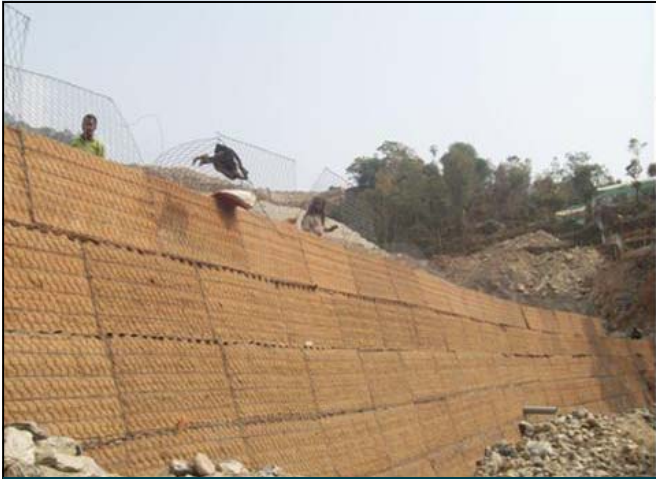
Green Terramesh soil reinforcement under construction
