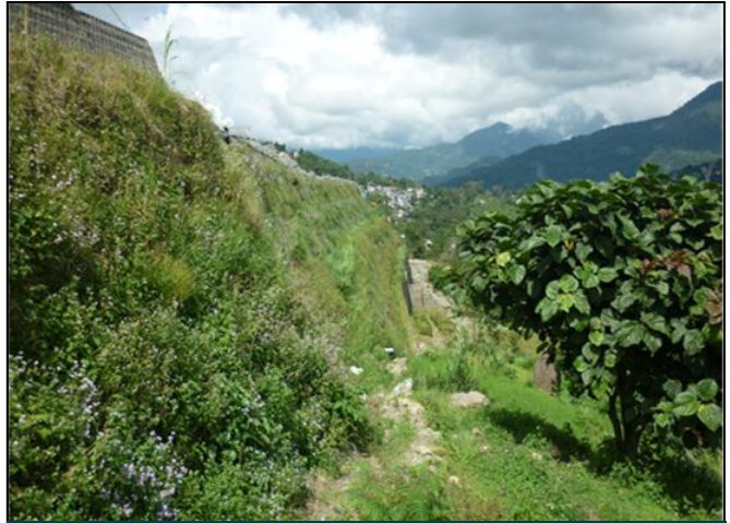
Green Terramesh soil reinforcement after vegetating
