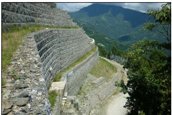
Main reinforced soil structure nearing full height
