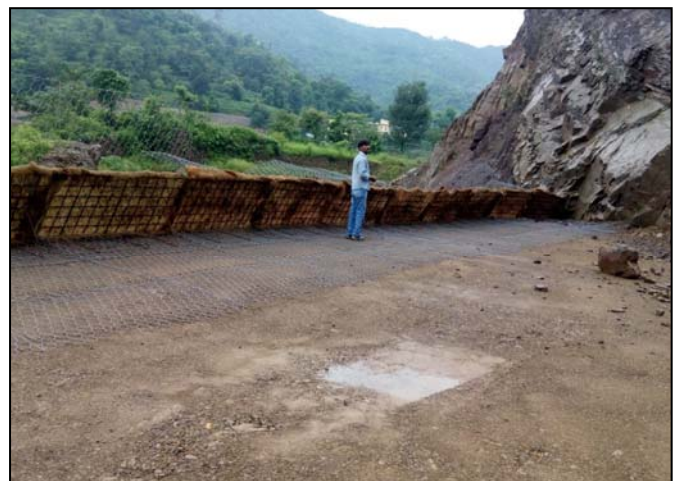
Green Terramesh units being placed, ready for backfilling
