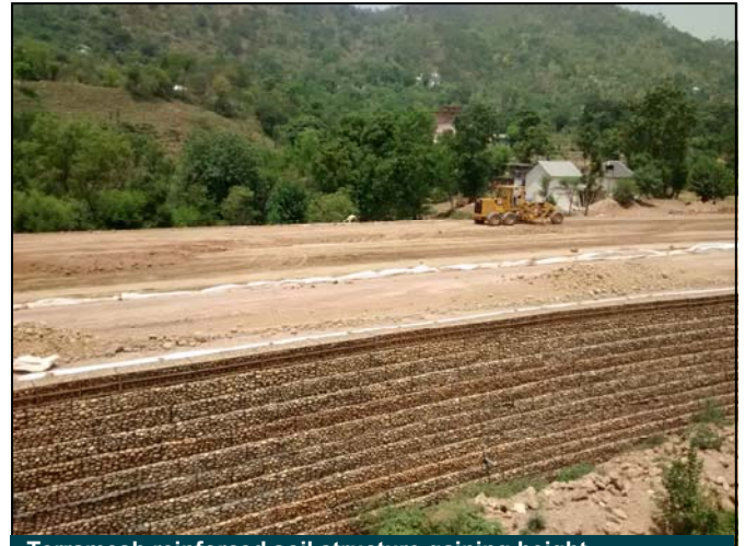
Terramesh reinforced soil structure gaining height
