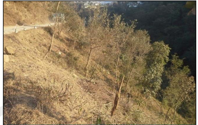
Existing highway, showing the downslope area
