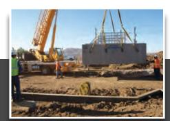
Low Pick Weights: Delivered in a top & bottom to minimize weight
