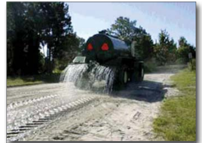
Figure 11. Water truck applying dissolved polymer flocculant
