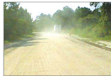
Figure 12. Road dust before applying polymer flocculant
