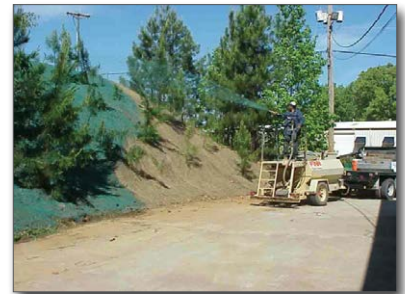
Figure 5. Hydroseeding the slope
