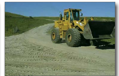
Figure 13. Road dust after applying polymer flocculant
