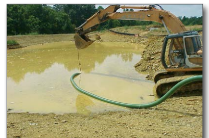
Figure 14. Sediment basin to be dewatered
