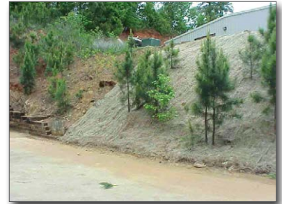
Figure 4. Slope covered with floc collection matting
