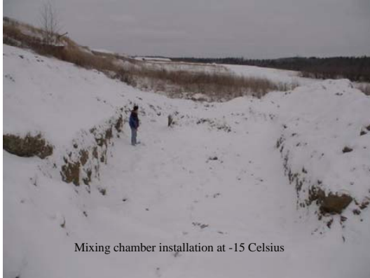
Figure 4: Mixing Chamber Excavation
