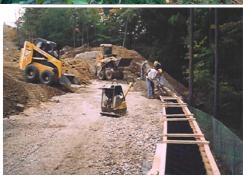
GEOSYNTHETIC DETAILS •Geoweb GW30V 6-inch, tan facia •Geogrid earth reinforcement layers
