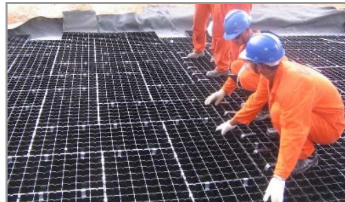
Figure 16: Connecting GEOTERRA™ Units
