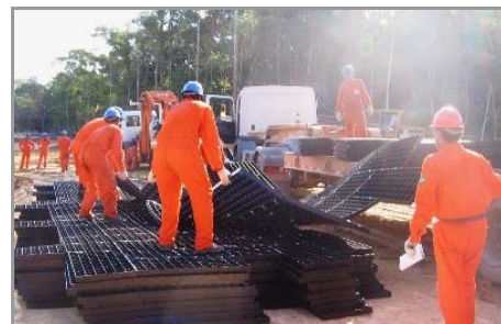
Figure 27: Transporting Pre-Assembled Mats from Off-Site
