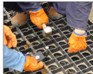
Figure 33: Driving the Anchor Head
