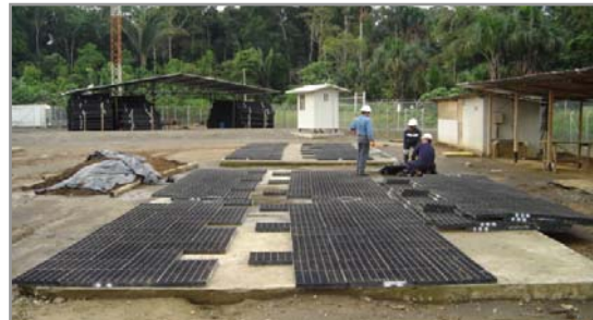
Figure 31: Connecting Pre-Assembled GEOTERRA™ Mats
