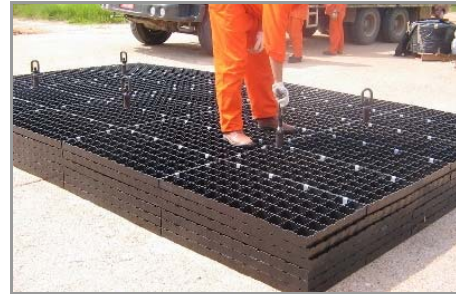
Figure 29: Assembling GEOTERRA™ Mats (Side-by-Side Pattern)
