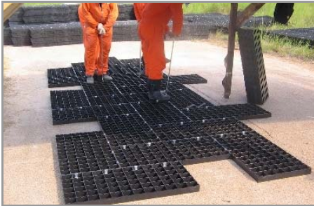
Figure 28: Assembling GEOTERRA™ Mats (Herringbone Pattern)
