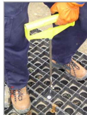
Figure 34: Setting the Earth Anchor
