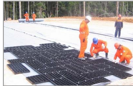
Figure 30: Placing GEOTERRA™ Mats Over Geotextile Layer
