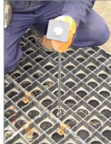
Figure 32: Installing the Earth Anchor
