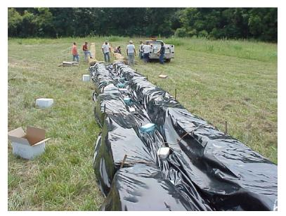
The site-specific Floc Logs are secured in the upper end of the treatment ditch.
