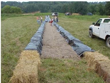
The lower part of the ditch is where the particle collection will take place. This is built wider than the mixing portion, to allow the water to slow its velocity.
