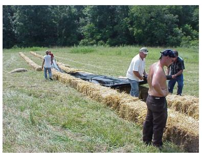
The ditch is lined with plastic sheeting to prevent erosion to the soil due to the high velocity flow expected.
