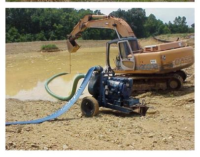
The pump is set up so that the feed is only pulling turbid water into the treatment ditch.
