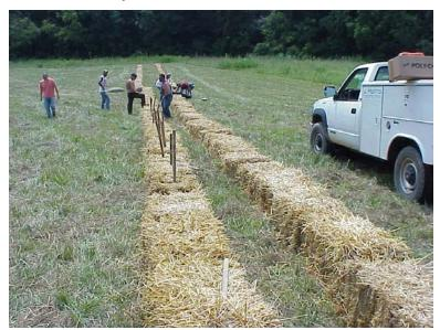
A ditch is built, using straw or hay bales, running downhill. The bales are staked down to hold them in place. The far end of the ditch is built wider; this is where the particle collection will occur
