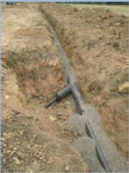
Methane Pipe Bedding/Seal
