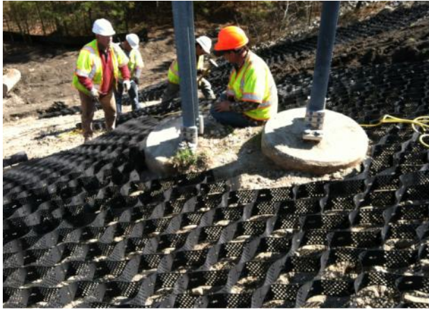
The flexibility of the GEOWEB system allows it to be placed around obstructions.
