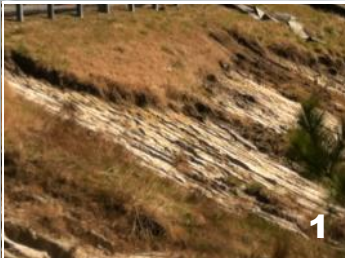
The flexibility of the GEOWEB system allows it to be placed around obstructions.
