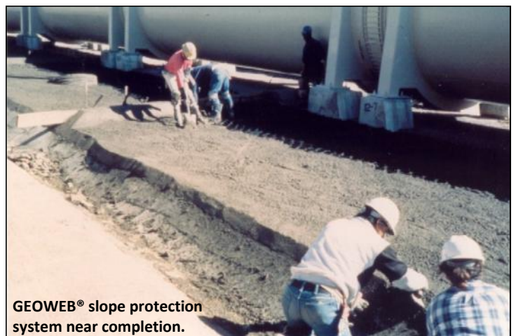
Spreading concrete within the GEOWEB® System
