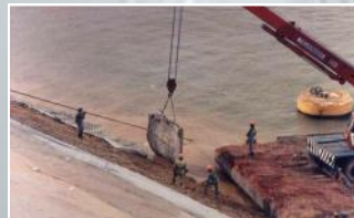
Top Left: Lifting the cured concrete filled GEOWEB sections with steel cables.
