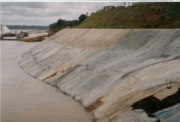
Bottom Photo: Completed concrete-infilled GEOWEB system covers the shoreline slope.
