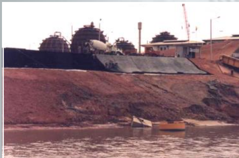
Installing concrete in the GEOWEB sections on the upper slopes.
