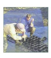
Anchors were evenly spaced and fastened over the tendons within the Geoweb sections to provide security against the stream's up-lift forces. During anchoring, the backhoe dropped crushed stone over the staked Geoweb sections. Equipment can be driven on the system as soon as the Geoweb cells are completely filled.
