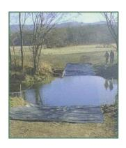
With the geotextile in place, one 16-foot edge of the Geoweb® system was placed geotextile the and over using anchored **ATRA®** anchors secured to the tendon ends. The Geoweb section was then stretched across the stream by pulling and expanding it to the opposite side of the stream.
