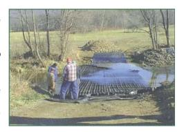
The Geoweb® system's side edges were placed in the predug trenches and anchored around the perimeter to hold the system in place. Anchors were driven with a hammer until the ATRA® Clip made contact with the streambed.
