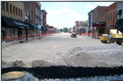
GEOWEB® system nearly filled with aggregate.
