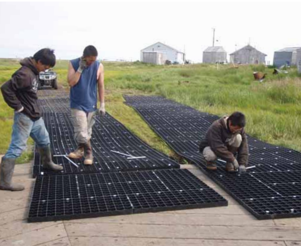
The trailbuilding units formed an interconnected structural mat pavement system.
