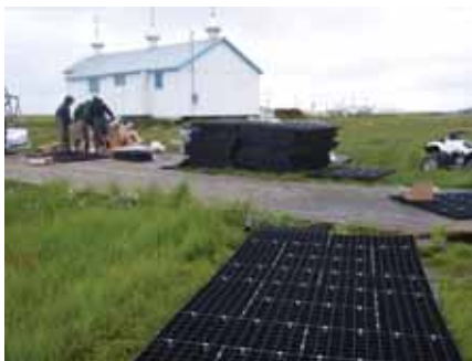
Moving pre-assembled 50-ft mat sections into position with ropes tied to ATVs.
