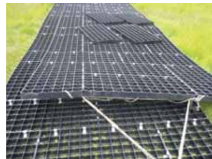
Moving pre-assembled 50-ft mat sections into position with ropes tied to ATVs.
