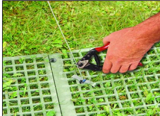
Figure 8. Cut the cable to loop the trailing end
