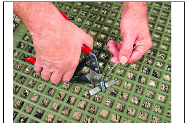
Figure 10. Cut the cable flush with the Gripple
