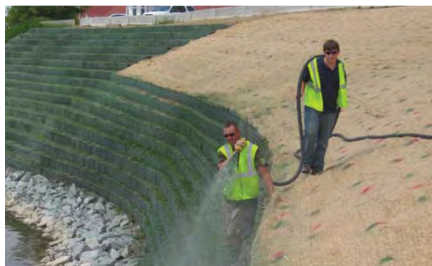
Tensar's HydraMax System can be installed three times faster than erosion control blankets with 1/3 of the man power.
