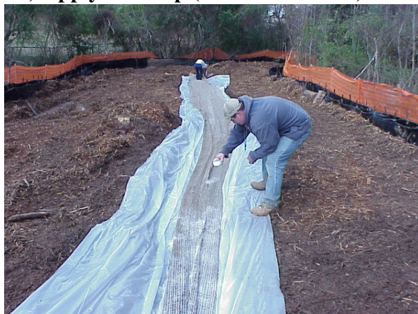
5) Apply Silt Stop (downstream end)
