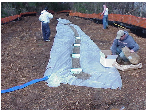
4) Place Floc Logs (upstream end)
